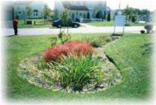
Figure 15: Bio-retention cells (also known as rain gardens) provide a storage area where storm water collects and filters into the soil, mimicking the site’s pre-development hydrology
